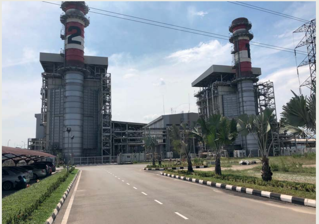
The combined cycle power plant in the city of Seberang Perai operates with an efficiency of more than 60 percent
